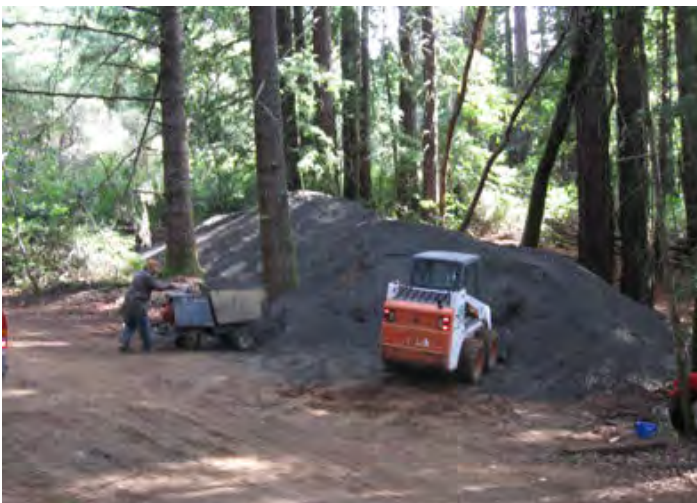
One of the four piles of base rock. The buggy can haul 2,000 pounds down the trail.
